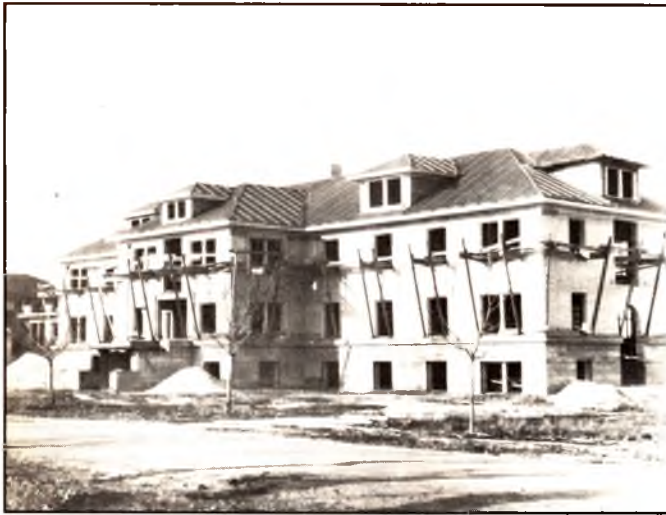
Samaritan Hospital in Nampa, Ida., under construction
