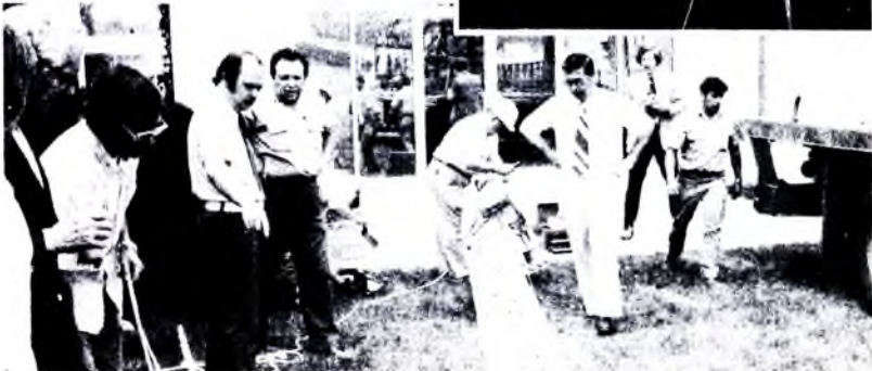
Spectators and specialists watched as the NARF radio tower was lifted by aerial crane to its rooftop position above the third floor of the General Board Building.
