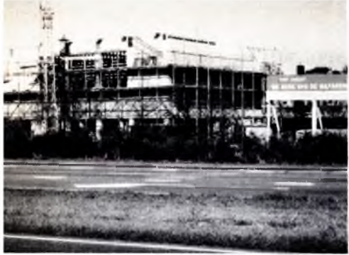
Haarlem, Holland church under construction.
