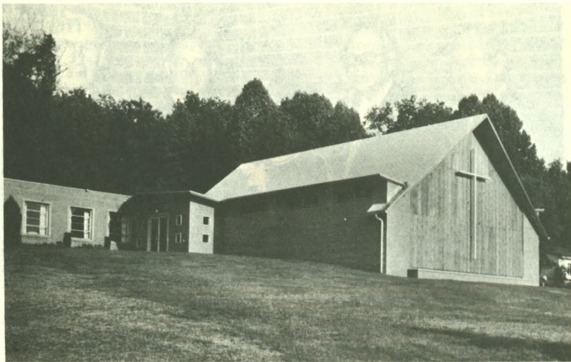
WEST AKRON (Ohio) Church dedicated its new sanctuary September 14 with Rev. Floyd O. Flemming, superintendent of the Akron District, as speaker. The building was designed by Mr. Donald Miller, Akron architect, and constructed by Mr. E. E. Riddle, contractor and builder from Tallmadge, Ohio. The property and building is valued at $85,000. The sanctuary will seat 225 and was designed and built for ease in future construction. Rev. Harvey L. Sprague is pastor.
