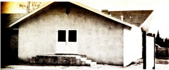
1 The completely remodeled McFarland, California, Church of the Nazarene, was dedicated by District Superintendent Eugene Stowe. Work on the project was done mostly on Saturdays by the men of the church, and in all took a little more than one year, at a cost for materials of about $10,000. Rev. Truman Duncan has been pastor since 1960.
