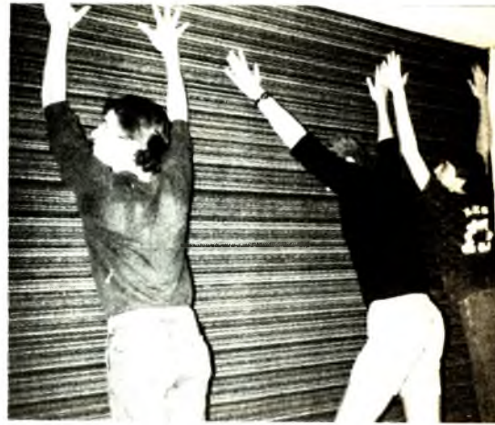
Applying the carpet to that same brick wall.
