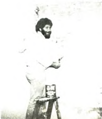
Kankakee, Ill., First Church youth pastor, Rev. Dave Clark, helps prepare for carpeting an old brick wall in a Sunday School room.
